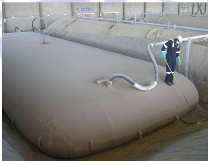
Image 5. Collapsible Fabric Fuel Tanks used for fuel storage throughout theatre.
