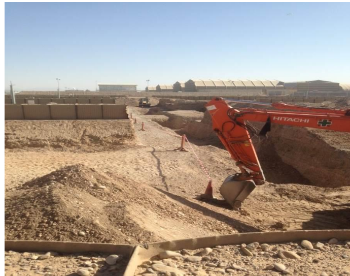
Image 6. Contaminated site at Kandahar undergoing excavation of the soil above 2000 ppm.
